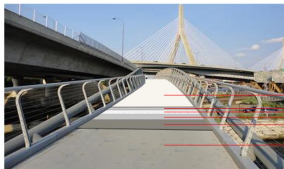
STARFLEX MONO TOP STARFLEX MONO TIX STARTEX NW / GM STARFLEX MONO TIX DUROGLASS FU RAPID CEMENT / DAMP SUBSTRATE
